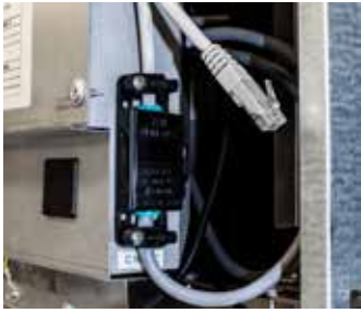
JUNCTION BOX AND CONNECTED ALARM CABLE (2.5 M) WITH RJ45 PLUG
