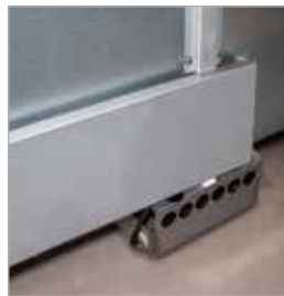
ELECTRICAL EVAPORATION OF DEFROST WATER
